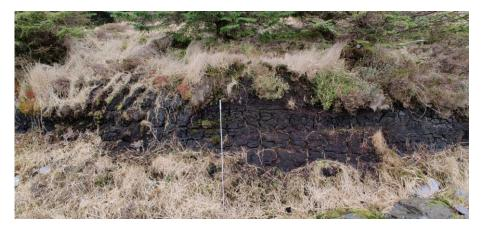
Figure 3-3: Compact peat side-cast along a track during previous construction works.
